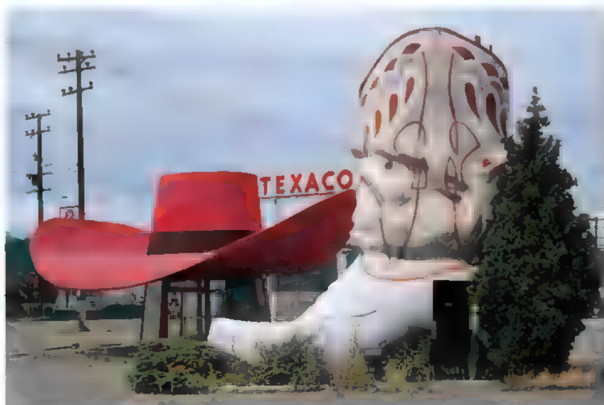
The builder of this 1955 Seattle, Washington, station patented his designs.
